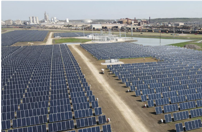
Solar Panels and Midlothian Industrial Unit
