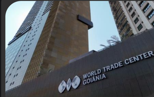
WTC Goiânia Commercial Building - GO
