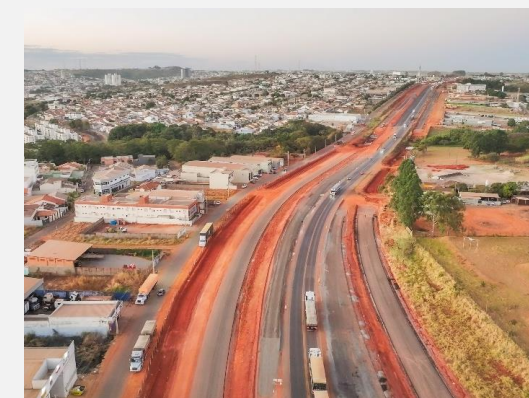
Eco050: Road widening Works in Catalão/GO
