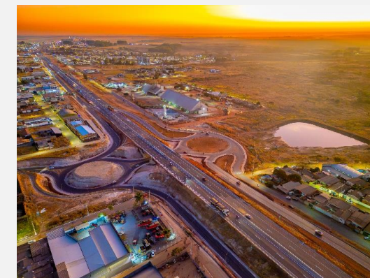
Eco050: Road widening in Cristalina/GO
