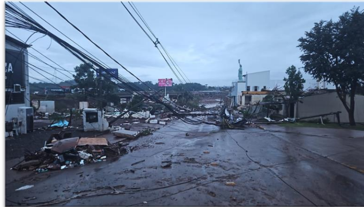
Internet network in Lajeado
