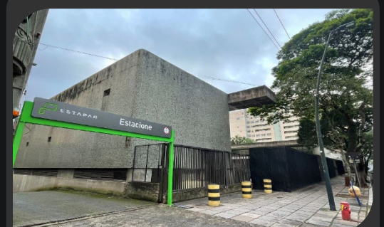
Duque Parking Building - RS
